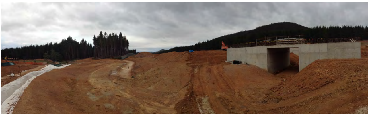
Underpass under construction, Majura Parkway May 2014
